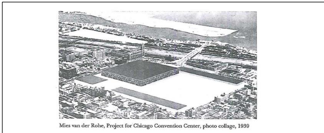
Figure 2.2: An Example of a Cleared Site. (The figure is from Burns, “On Site: Architectural Preoccupations,” 152.)
